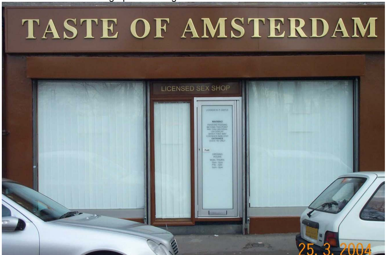
Photograph of frontage of 437 Millbrook Road West
